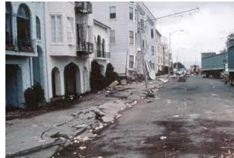
Liquefaction
